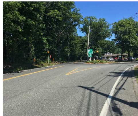
North Road at Chelmsford Road looking north.
